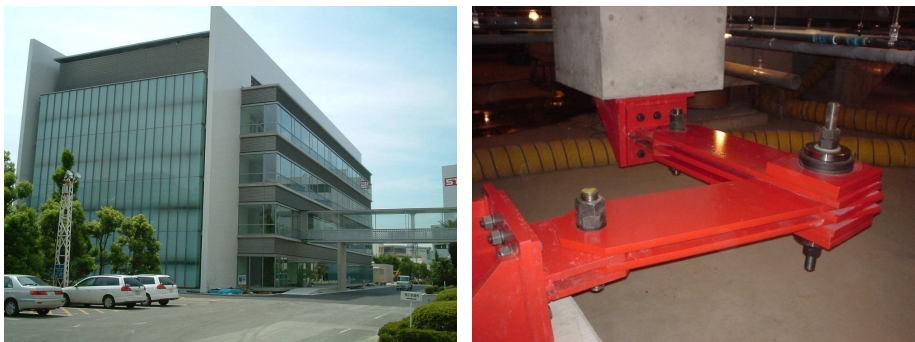
Fig. 9. Five-storey building in Japan with base isolation incorporating RFDs
