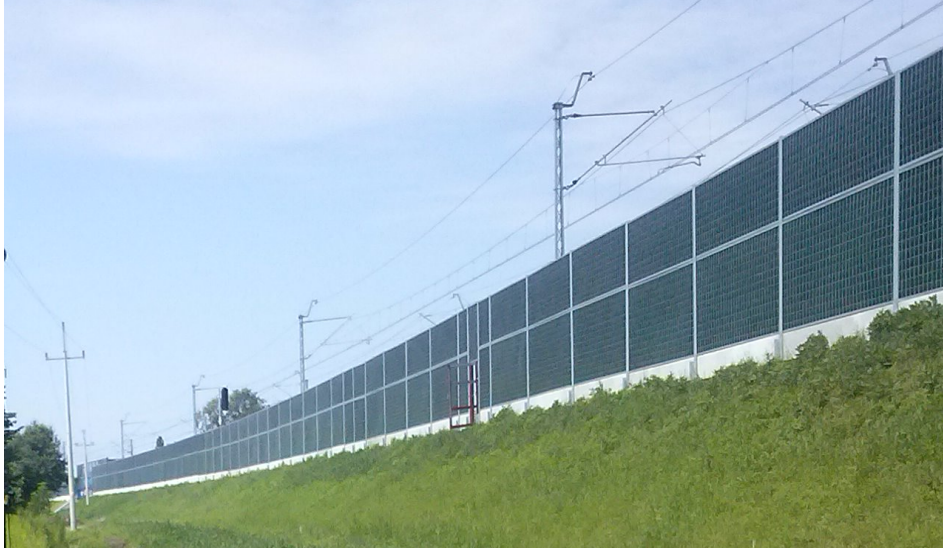
Fig. 2. Noise barrier view (in the direction of Dębica)
