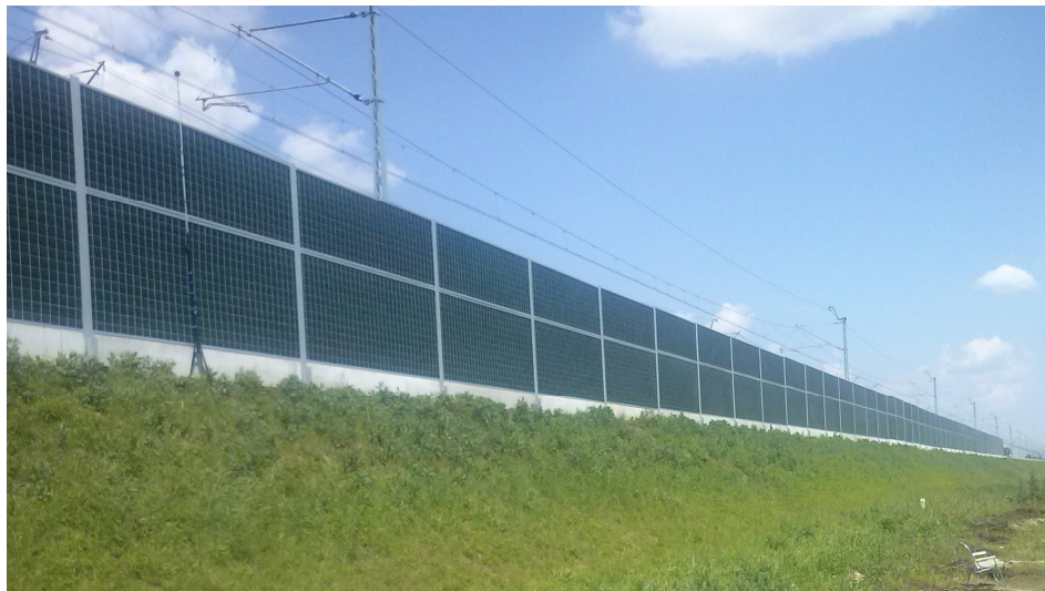
Fig. 1. Noise barrier view (in the direction of Rzeszów)
