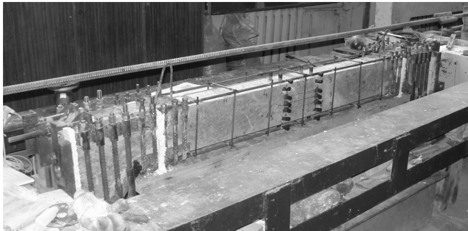
Fig. 4. Installation of jacketing reinforcement
