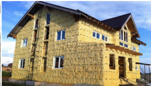
Fig. 9. Polyurethane foam insulation
