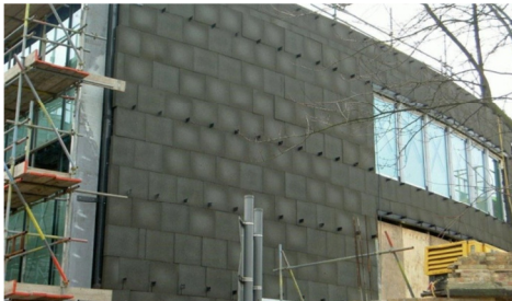
Fig. 8. Foam glass insulation
