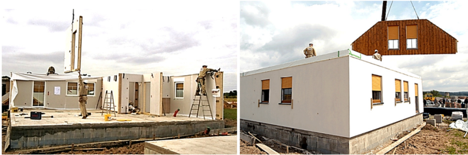
Fig. 2. Construction of panel construction system [12]
