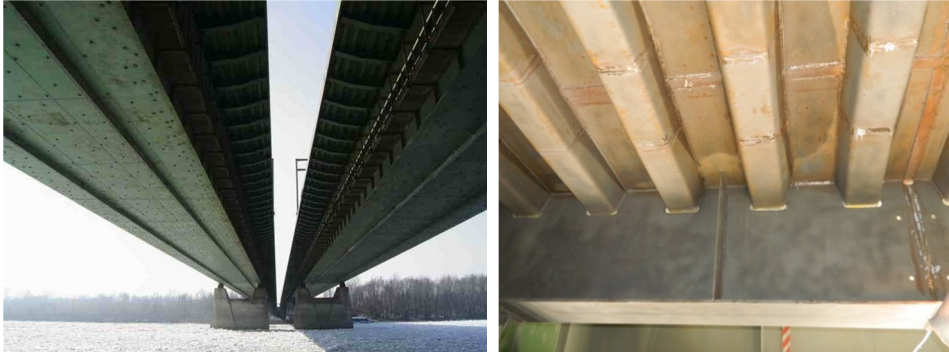
Fig. 1. The Grot-Rowecki Bridge: general view of box girders (left), the orthotropic deck (right)
