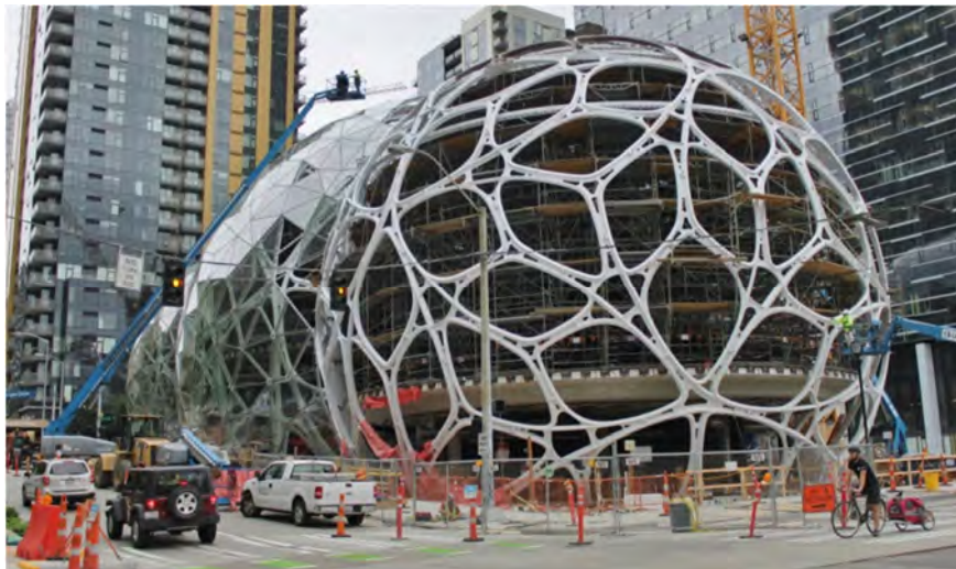
Fig. 6. Amazon Spheres – spherical conservatories serve as employee lounge and workspace located on the headquarters campus of Amazon company in Seattle, USA, completed in January 2018: steel structure under construction (author of photography: SounderBruce [9])
