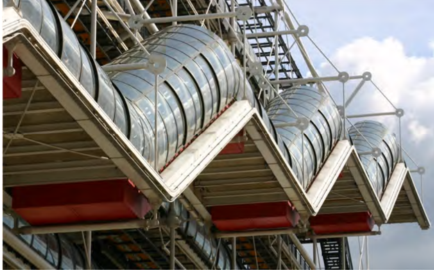
Fig. 9. Centre Georges Pompidou, Paris, France. Visible enlarged gusset plates, additionally accentuated by the central hole (author of photography: V C [10])
