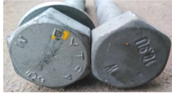
Fig. 2. Bolts in analysed joint: 1–old bolt, 2–new bolt bought in Poland
