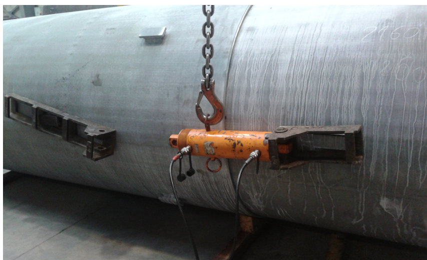
Fig. 1. Assembly of the steel shell tower trunk
