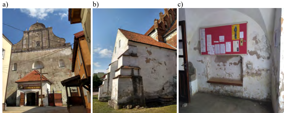
Fig. 1. St. Andrew's church in Barczewo - a) main entrance b) damaged side elevation c) multiple traces of damp visible on the walls from the inside
