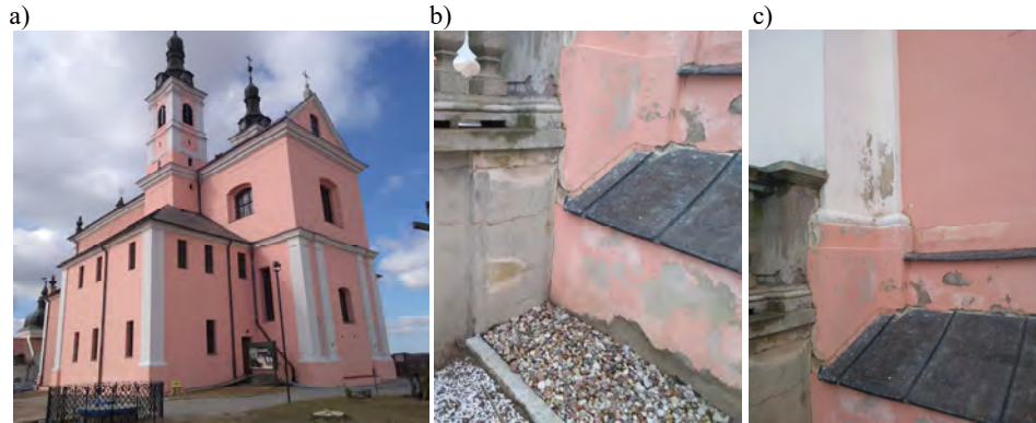
Fig. 3. A church under the invocation of St. Mary's Immaculate Conception - Wigry, a) general view of the building complex b) and c) visible outer layer damage caused by damp
